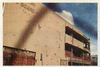
Frag marks in south side of Oklahoma Water Resources Board building (across 5th street from blast) indicate power of blast and velocity of fragments.
